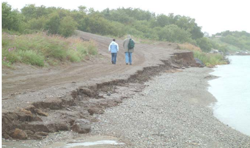
Photo 2: Erosion by the lake, July 2004.
